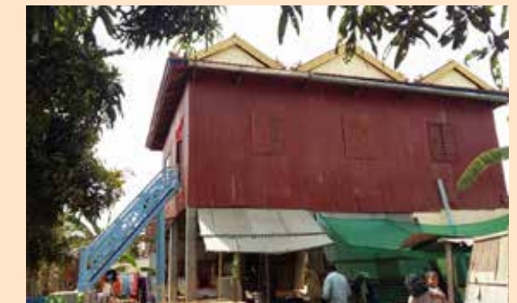
Mrs. Sa En's new 6m by 9m, two-story house.
