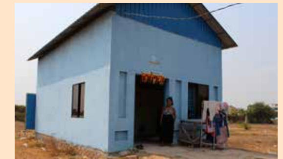
Mrs. Sreymom in front of her new concrete house.
